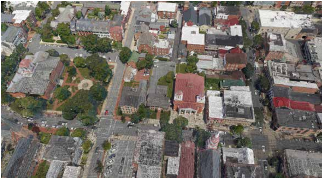
Figure 2. 3D city view of Frederick, MD using 2cm nadir and 3cm GSD oblique imagery collected by Icaros, Inc. This imagery is converted to a texture map and then reconstructed on to the 3D model of the city through an automated process. The above image is a wireframe rendering of the model with texture applied.
